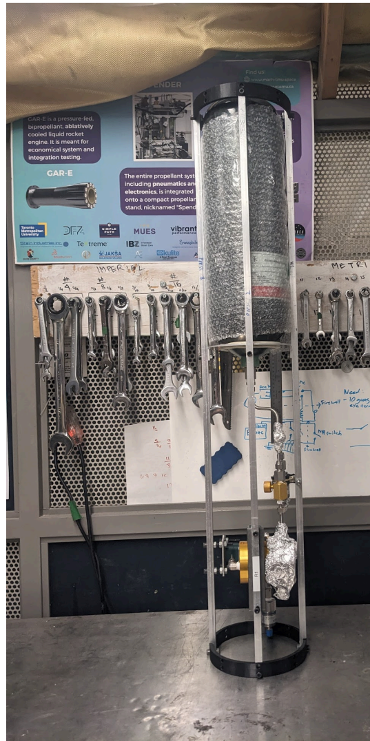
Figure 5.1.1.1.3: Completed pressurant bay plumbing
