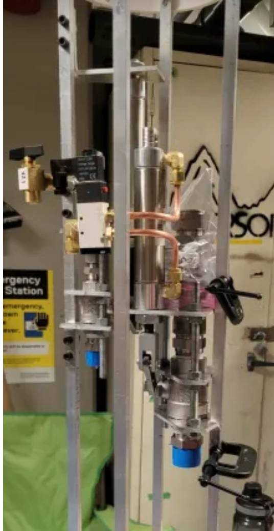
Figure 5.1.2.2.1: Run bay with installed MOV and MFV assemblies.
